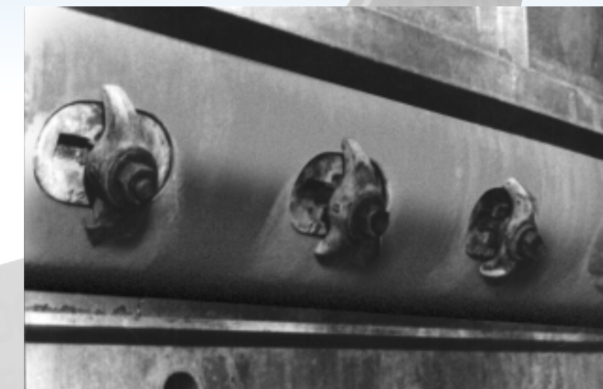
...INSTALL TOPOG-E GASKETS!
